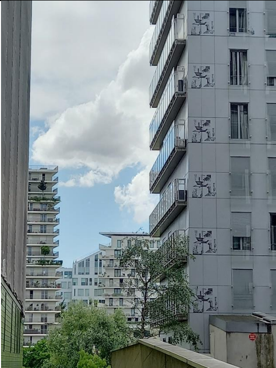
Figure 128 E5 building, thickness of the building. Balconies. Source M. Apostolou
