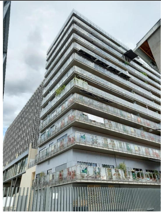
Figure 129 E5 building, thickness of the building. Balconies. Source M. Apostolou
