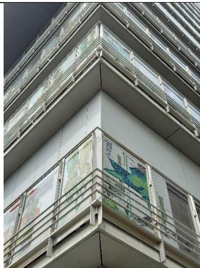
Figure 137 E5 building, detail façade. Source M. Apostolou
