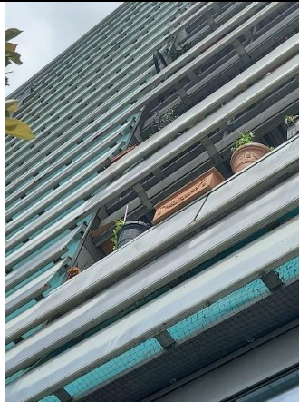
Figure 70 This cladding is made of coloured and translucent polycarbonate panels with three different levels of transparency. The panels are fixed on a secondary aluminium frame that houses the panel support connectors, which were specifically designed for this project, to allow the panels to be installed inclined, usually arranged horizontally or vertically. A coloured breathable membrane is placed in front of the insulation to protect it from rain and to provide a coloured background so as to increase the colour effect of the cladding. Source M. Apostolou
