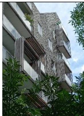
Figure 104 Details, façade. Openings and balconies. Source M. Apostolou
