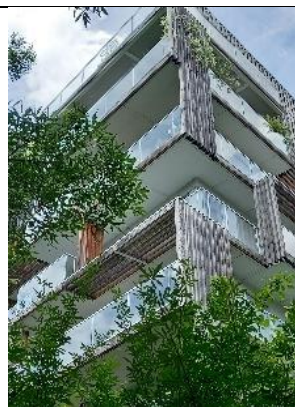
Figure 103 Details, façade. Openings and balconies. Source M. Apostolou
