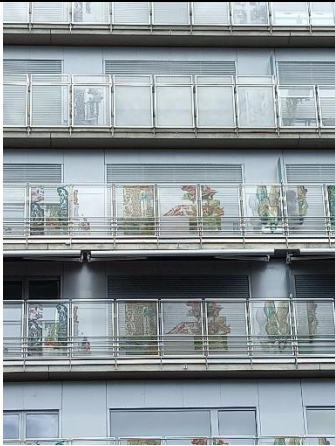
Figure 133 E5 building, detail openings south façade. Source M. Apostolou
