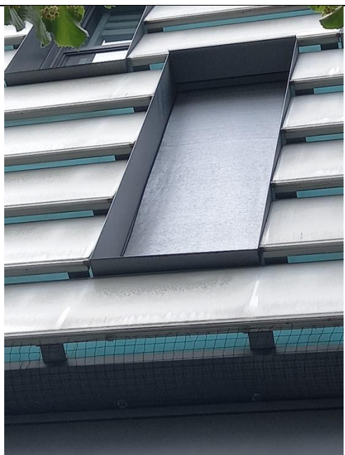
Figure 53 Façade, detail. Building E1. Source M. Apostolou
