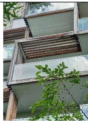
Figure 105 Details, façade. Openings and balconies. Source M. Apostolou
