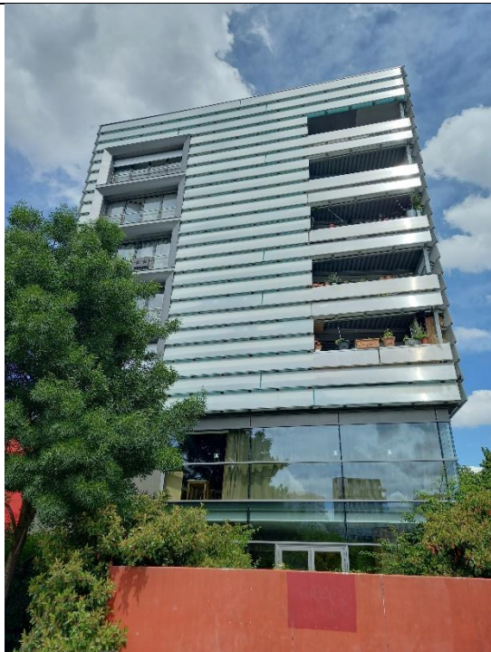
Figure 42 Building E1, view from the parc, façade. Source M. Apostolou
