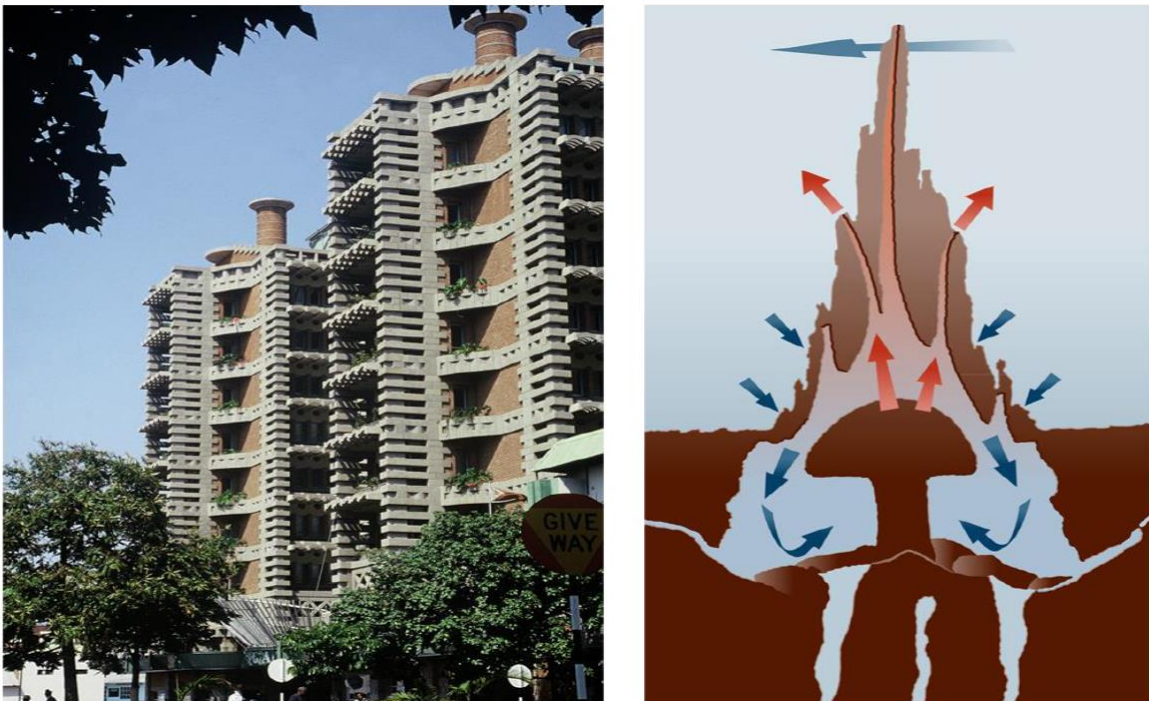
Figure 7 - Eastgate center (left) and ventilation principles based on termite mound (right) (Okeke et al., 2019)
