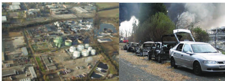
Figure 1.6 – Aerial view of the devastation after the Buncefield accident.
