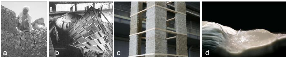
Figure 2.5 Applications of wet sand in architecture. (a) conglomeration of sand and salt in Siwa oasis in Egypt [111] (b) sand formwork for concrete casting in Philips pavilion by Le Corbusier [112] (c) reinforced sand tower, CRATERRE laboratory (d) accumulation of sand by wave forces, Growing Islands project by Self-Assembly lab [113]
