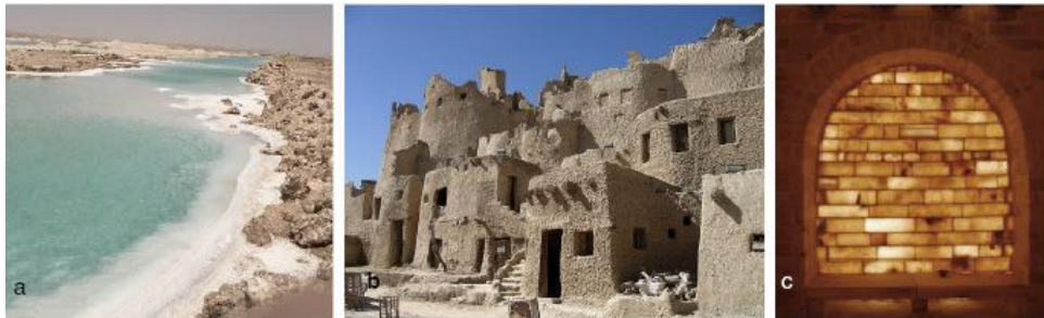
Figure 2.15 Salt architecture in Siwa, Egypt. (a) salt lakes (b) houses with sand and salt mortar (c) salt bricks
