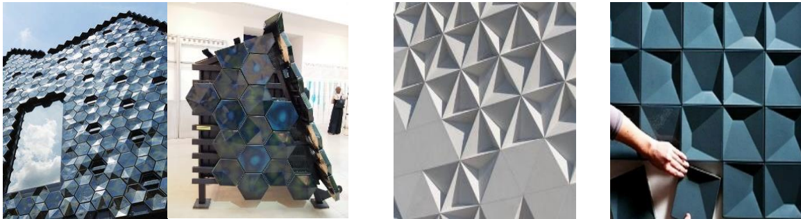
Figure 6.30 Standard 3D tiles are used for the exterior cladding of der Kulturen museum in Basel (left), Liverpool department Store in Querétaro City (middle) and for interior cladding (right)
