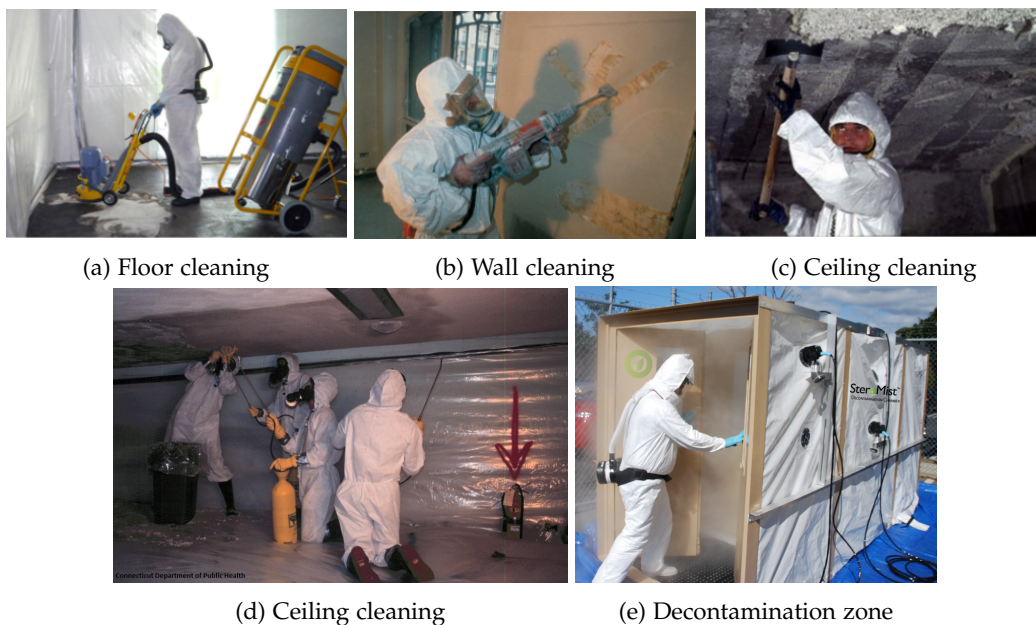
Figure 1.5: Different scenarios of asbestos cleaning process
