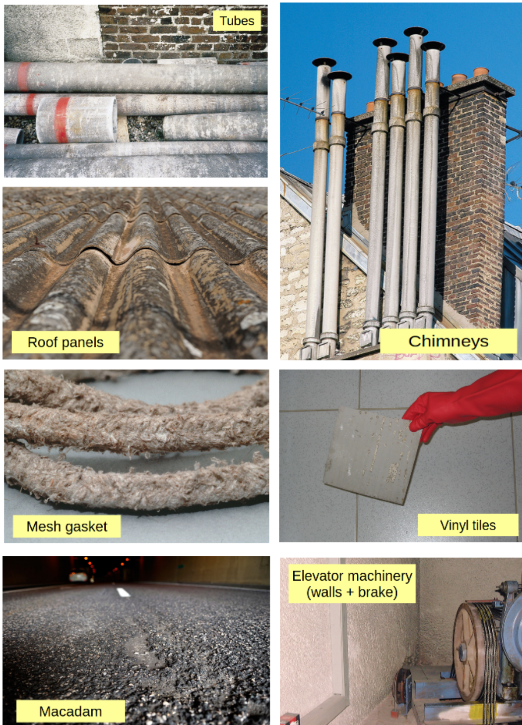
Figure 1.2: Presence of asbestos contamination inside residence-B
