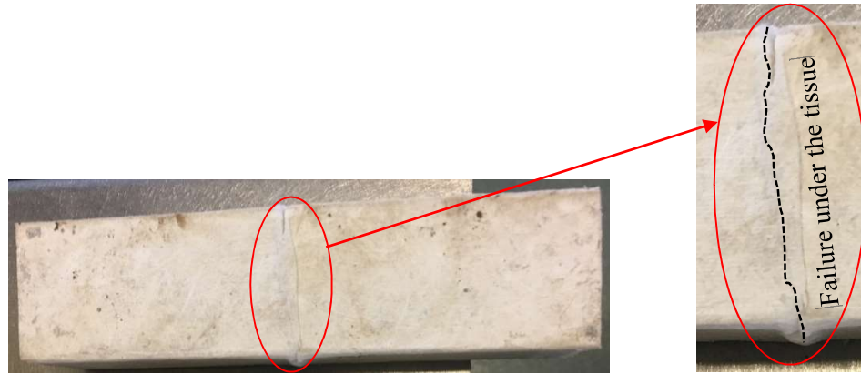
Figure 5- 11: Cracking patterns of beam (3-Sides)
