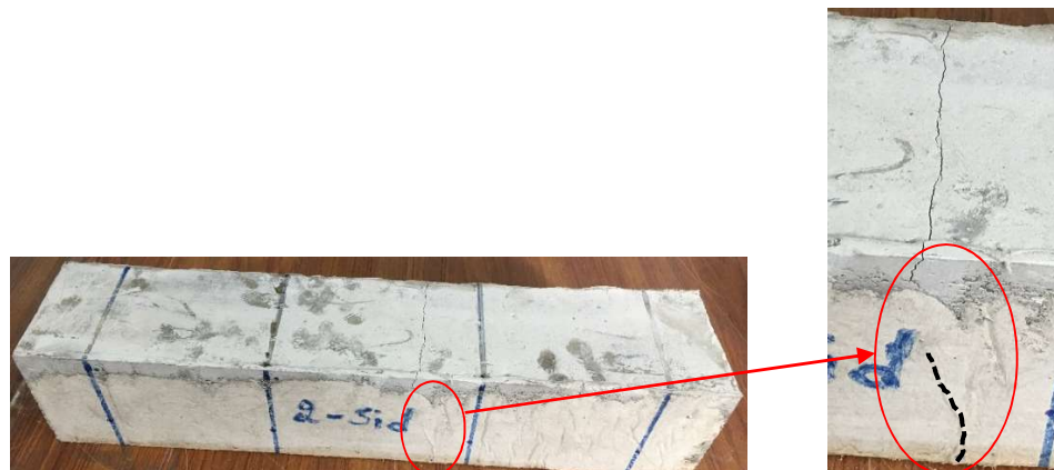
Figure 5- 10: Cracking patterns of beam (2-Sides)
