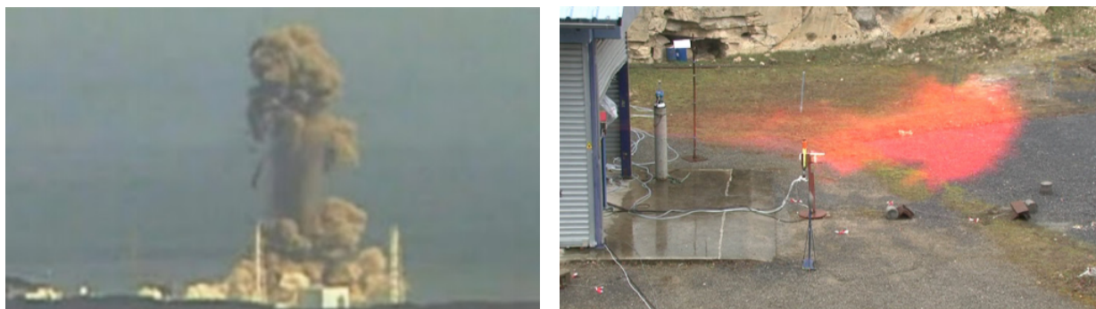
(a) Explosion of Fukushima reactor 3
