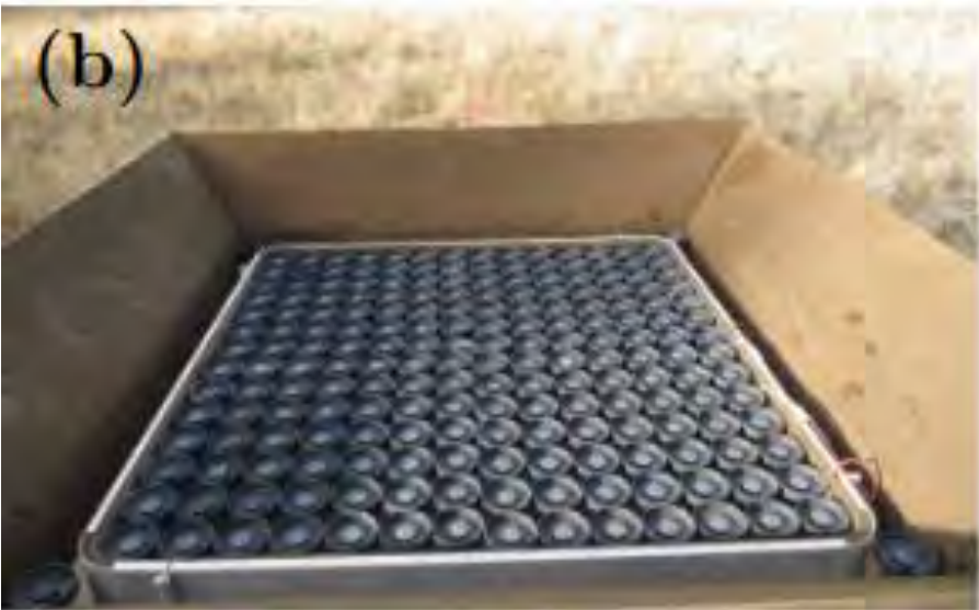
Figure A1.8: Sodar1 installation close-up photo.
