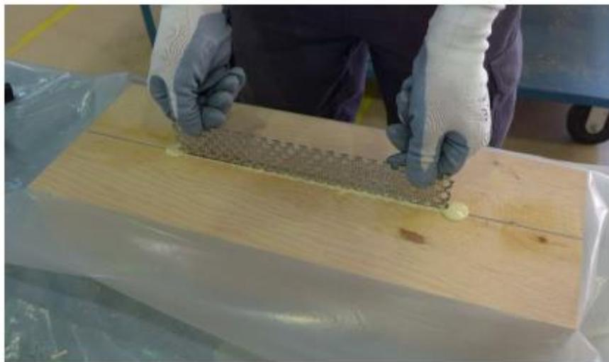
Figure 1.8. HBV installation, by Gerber [59]
