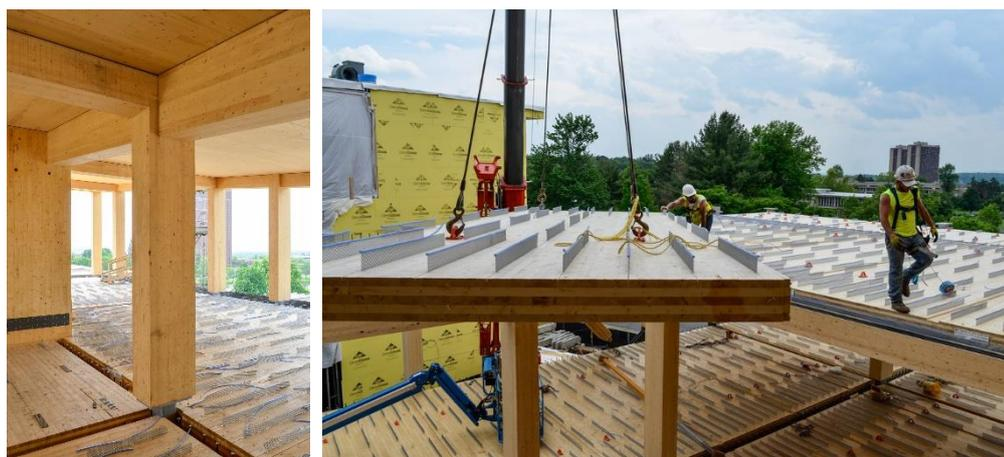
Figure 1.1. CLT panels with preinstalled HBV connectors, at the UMass Olver Design Building, University of Massachusetts, Amherst, USA. Image courtesy of Alex Schreyer.
