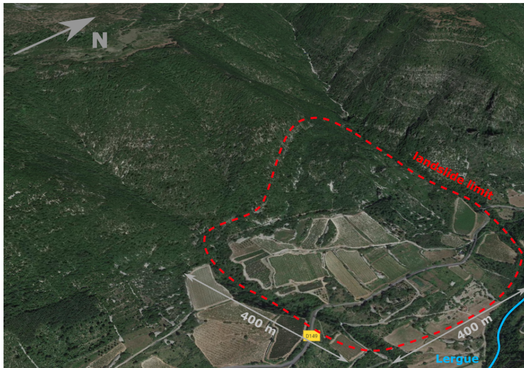
Figure 5.2: Aerial view of the Lodève landslide (Google Earth satellite image)
