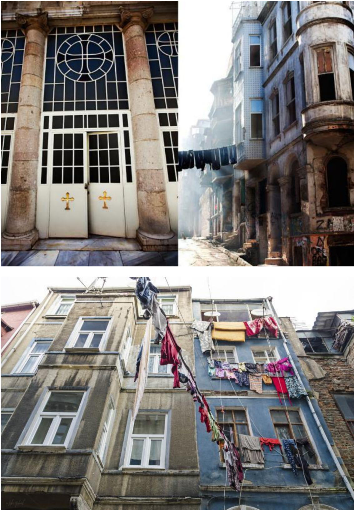
Figure 6.7 (a) (b) A typical building in Tarlabasi (Author's photography)
