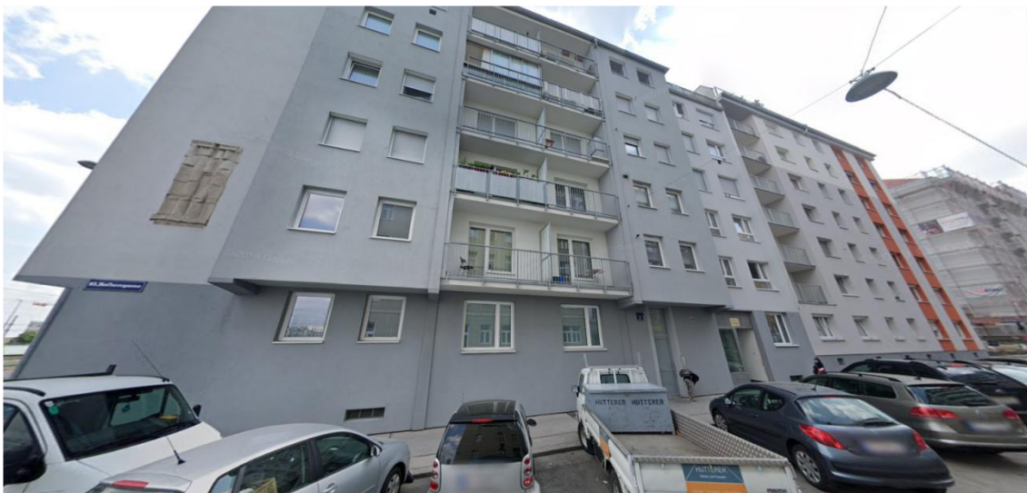
Figure 8.21 Kretaviertel building - Quality "4" (Taken from Google Earth)
