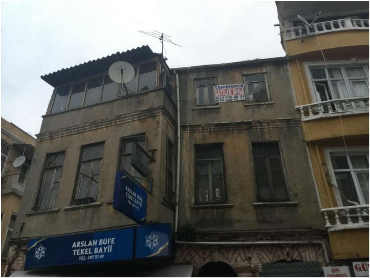
Figure 8.3 Tarlabasi building - Quality "1" (Photographed by the author)
