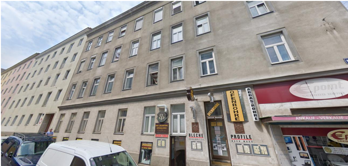
Figure 8.19 Kretaviertel building - Quality "2" (Taken from Google Earth)
