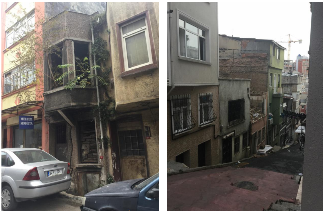
Figure 8.2 (a) (b) Tarlabasi building - Quality "0" (Photographed by the author)
