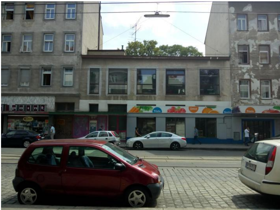
Figure 6.13 Typical worn down building in Kretaviertel (Author's photography)
