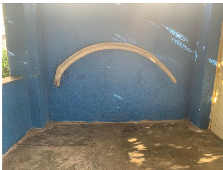
Figure 149 - The wood piece fixed to the wall
