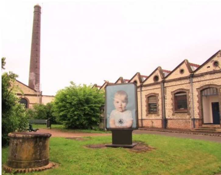
FIGURE 1.13 – L’usine St Joseph de Troyes
