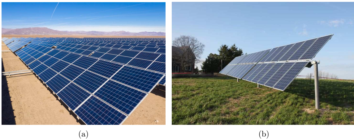
Figure 1.3: (a) A fixed-tilt flat plan PV plant [4], (b) a single-axis tracking plant [5].
