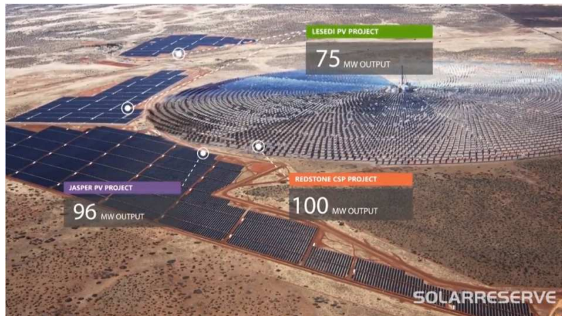
Figure 1.21: South-Africa’s largest renewable energy project Redstone CSP project, adjacent to the 75 MW and 96 MW PV solar power projects successfully developed and implemented by SolarReserve [27].
