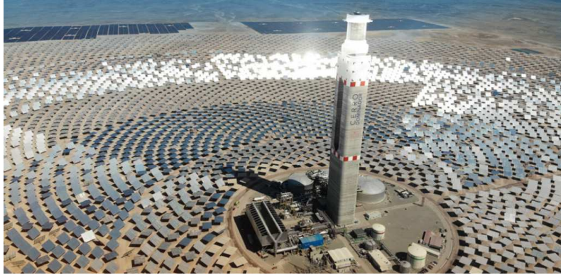
Figure 3: Cerro Dominador non-compact PV-CSP hybrid plant located in Northern Chile with a peak power of 210 MW [2].
