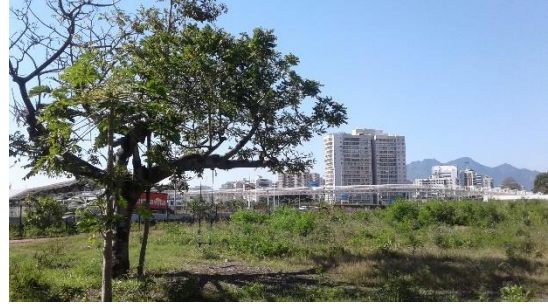
Figure A16: Passerelle du BRT Vila Autódromo
