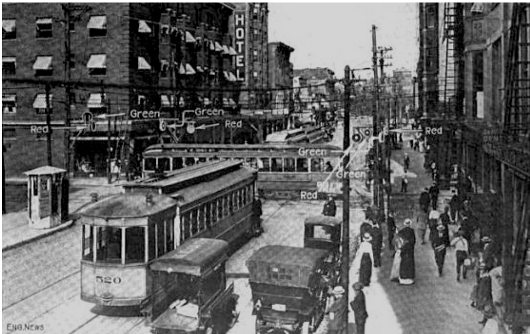
Figure 2.1: The First Modern Traffic Light Control System, Installed on Euclid and 105th Avenue. Cleveland, Ohio, August 1914.
