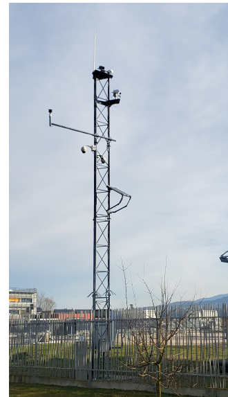
(d) Pole for meteorological conditions measurement at CEA-INES.
