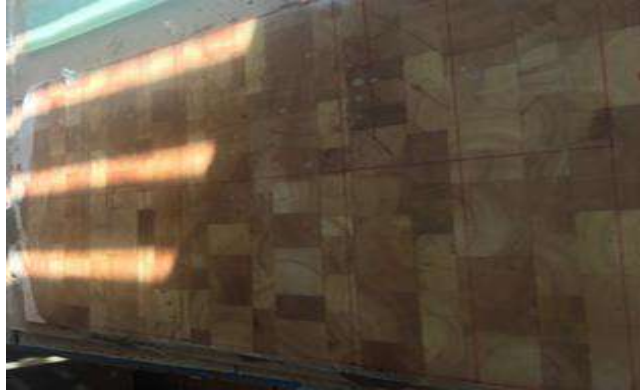
(a) The first fully wet GFRP ply and balsa panel.
