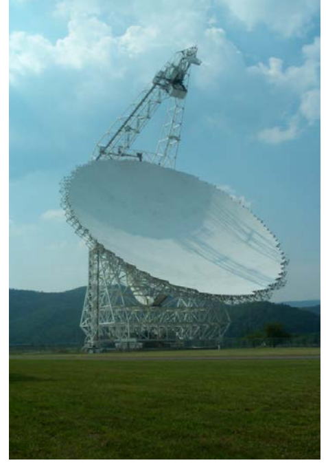
Figure II.5: Green Bank Telescope 100-m, de 1 à 100 GHz.
