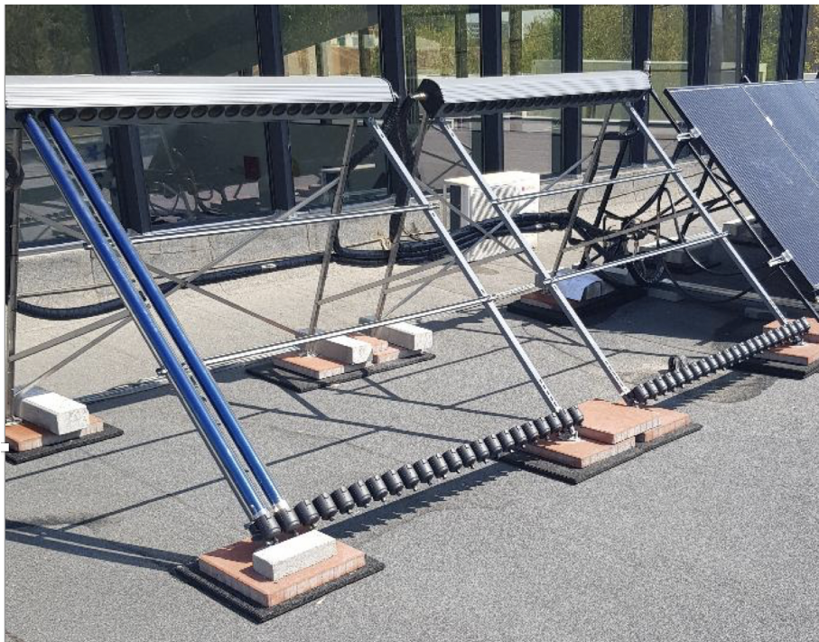
FIGURE 5.8: Photography of the solar thermal panels before installing the evacuated tubes
