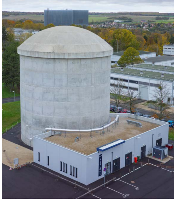
Figure 4.1: Aerial view of VeRCoRs mock up - EDF Lab Les Renardières. ©EDF
