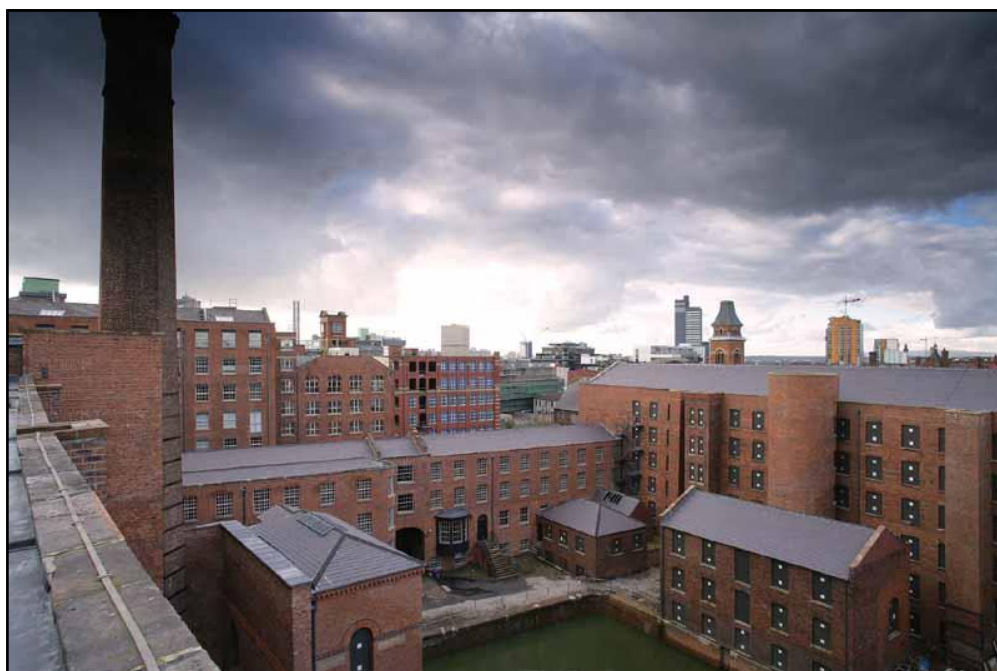
Figure 129 : Murrays' Mill , Manchester (Ancoats) 559
