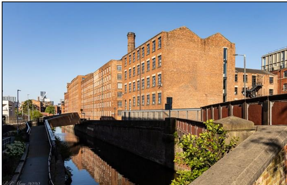
Figure 128 : Murrays' Mill , Manchester (Ancoats) 558
