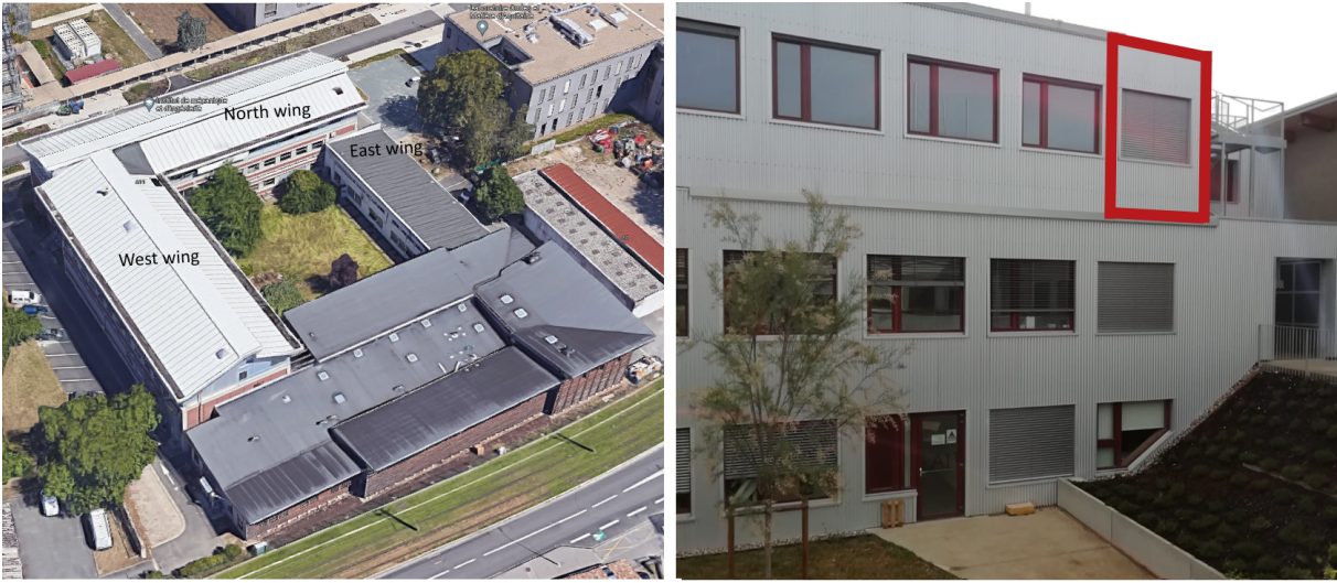
Figure 6.42 – Google image of A11 building (left) and view of the tested office (in red) west facade from the central building area (right).
