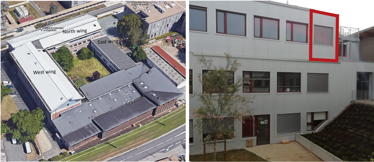
Figure 6.42 – Google image of A11 building (left) and view of the tested office (in red) west facade from the central building area (right).
