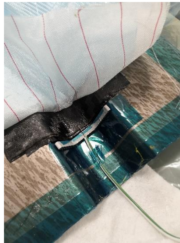
Fig. 2. 8. Thermocouples installation for temperature tracking during curing
