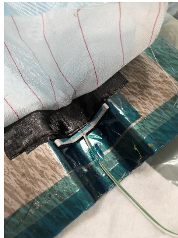
Fig. 2. 8. Thermocouples installation for temperature tracking during curing
