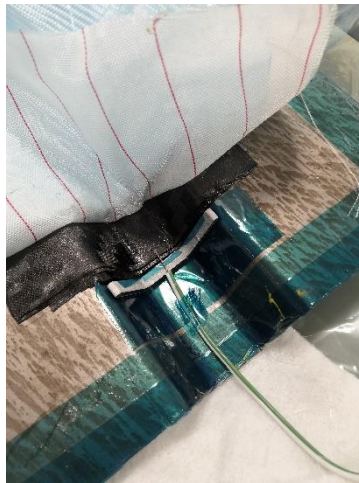
Fig. 2. 8. Thermocouples installation for temperature tracking during curing
