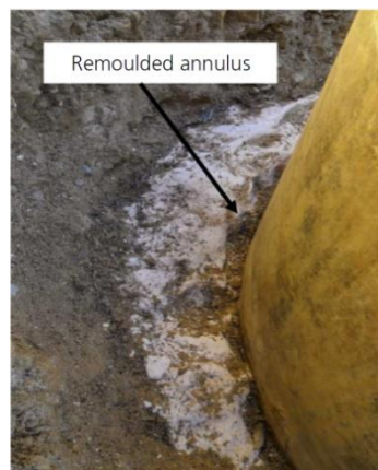
Figure 1.17 : Side view of a pile after being driven in low to medium density chalk, (Ciavaglia et al. 2017)
