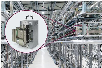
(b) Valve building: HB-SMs assembly. Source: [50].
