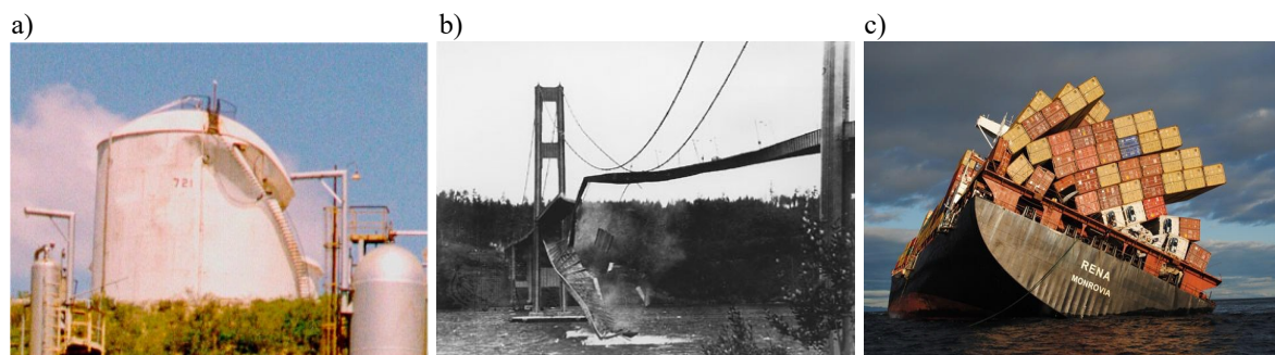
Figure 2: Examples of the risk of instabilities a) Buckling of liquid storage tanks under uni-form pressure at Penuelas, Puerto Rico. Image credit: Luis A. Godoy [7]. b) Collapsing of the Tacoma Narrows bridge due to strong winds. Image credit: The United State Government, retrieved from the data of the 7 th of November 1940. c) MV Rena cargo ship broken in half and loss of containers due to the periodicity and high amplitude of the waves. Image credit: Maritime New Zealand.
