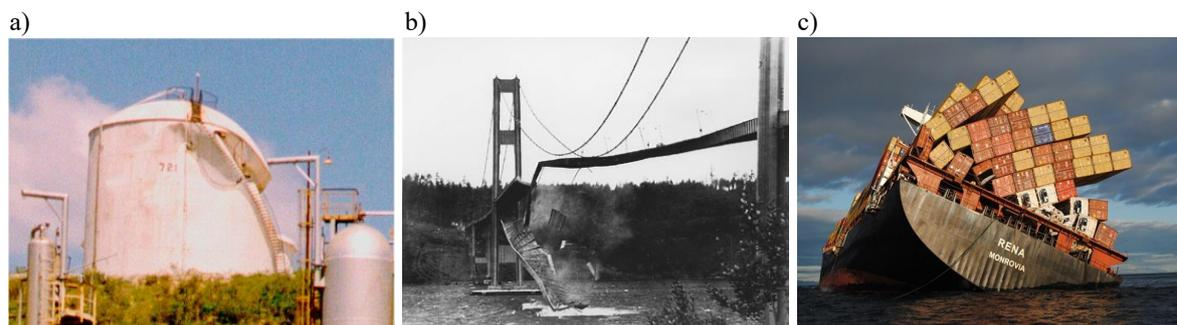
**Figure 2:** Examples of the risk of instabilities a) Buckling of liquid storage tanks under uniform pressure at Penuelas, Puerto Rico. Image credit: Luis A. Godoy [7]. b) Collapsing of the Tacoma Narrows bridge due to strong winds. Image credit: The United State Government, retrieved from the data of the 7<sup>th</sup> of November 1940. c) MV Rena cargo ship broken in half and loss of containers due to the periodicity and high amplitude of the waves. Image credit: Maritime New Zealand.
