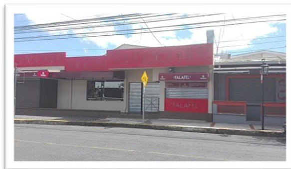
Image 248 Non-accessible entrance and take-out window
