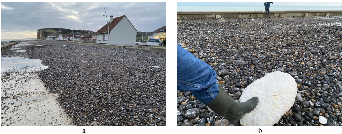
Figure 20 - Washover sediment found on top of the seawall of Hautot-sur-Mer after Storm Ciara on 2020/02/14 (Credit: A. Soloy, 2020)
