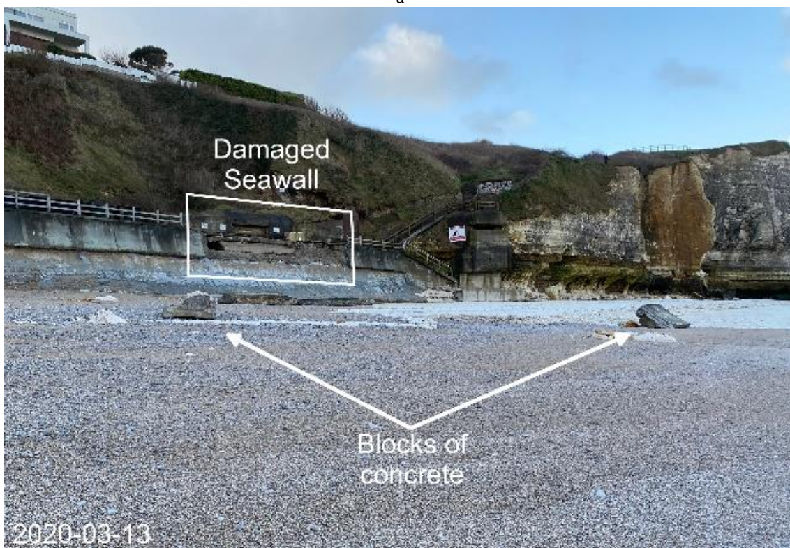
Figure 68 – a: Photograph taken on 2019/12/13 (Storm 5) in Etretat showing the overtopping of waves over the seawall (Département de Seine-Maritime, (ROL, 2019)) ; b: Seawall damages observed in Etretat on 2020/03/12 after a storm event.
