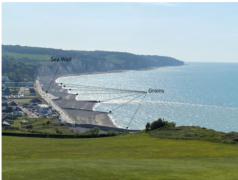
Figure 14 - Typical coastal defense structures encountered on the beaches of Normandy. Photography taken at mid- to high tide in Hautot-sur-Mer (credit: J. Steele, 2021).
