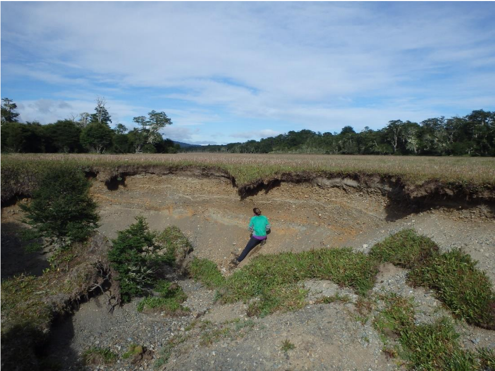
Photo 5 Trench near Puesto La Quesaria -54.52300 -67.04391
