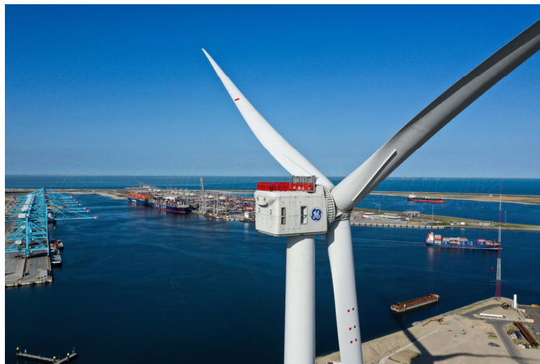
Fig. III-6 GE Haliade-X 14 MW offshore wind turbine prototype [169].
