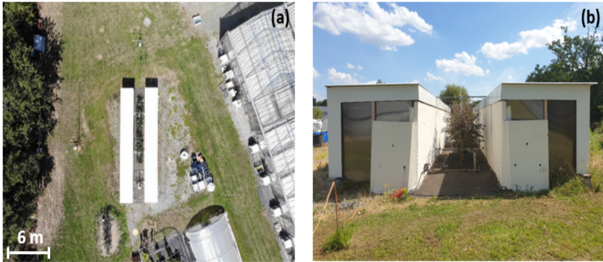
FIGURE 33 – Canyon street at 1/5 scale built at Institut Agro, in Angers (France). (a) : top view, (b) : front view Photo credit : INRAE, OPAALE research unit.
