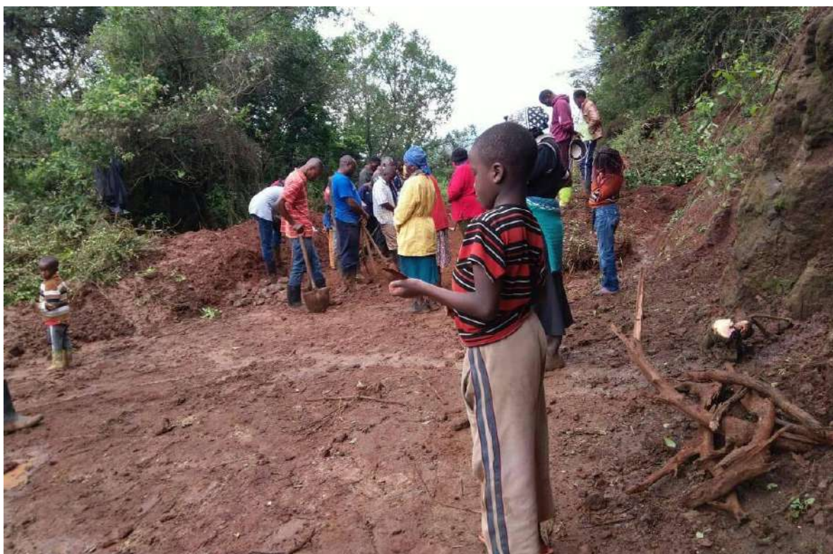
Figure 4.28: Joint action by residents to clear a section of a road blocked by a landslide.
