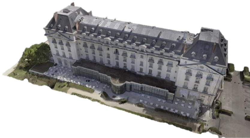
Figure A.1 3D reconstruction using drone photogrammetry [Dron00]
