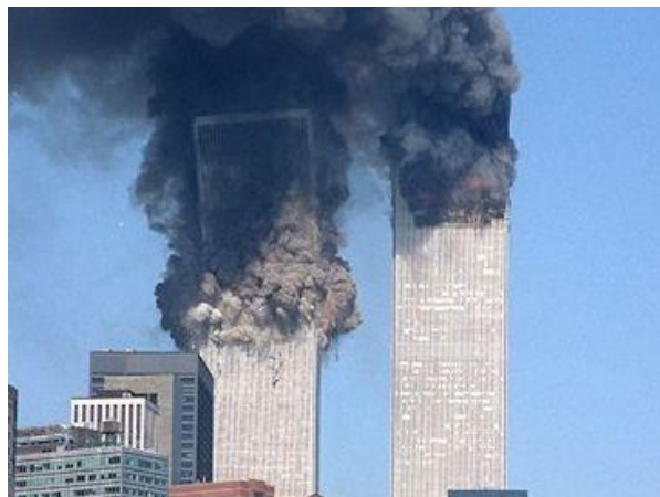
Figure 1 World Trade Center collapse, 11 September 2001 [2]
