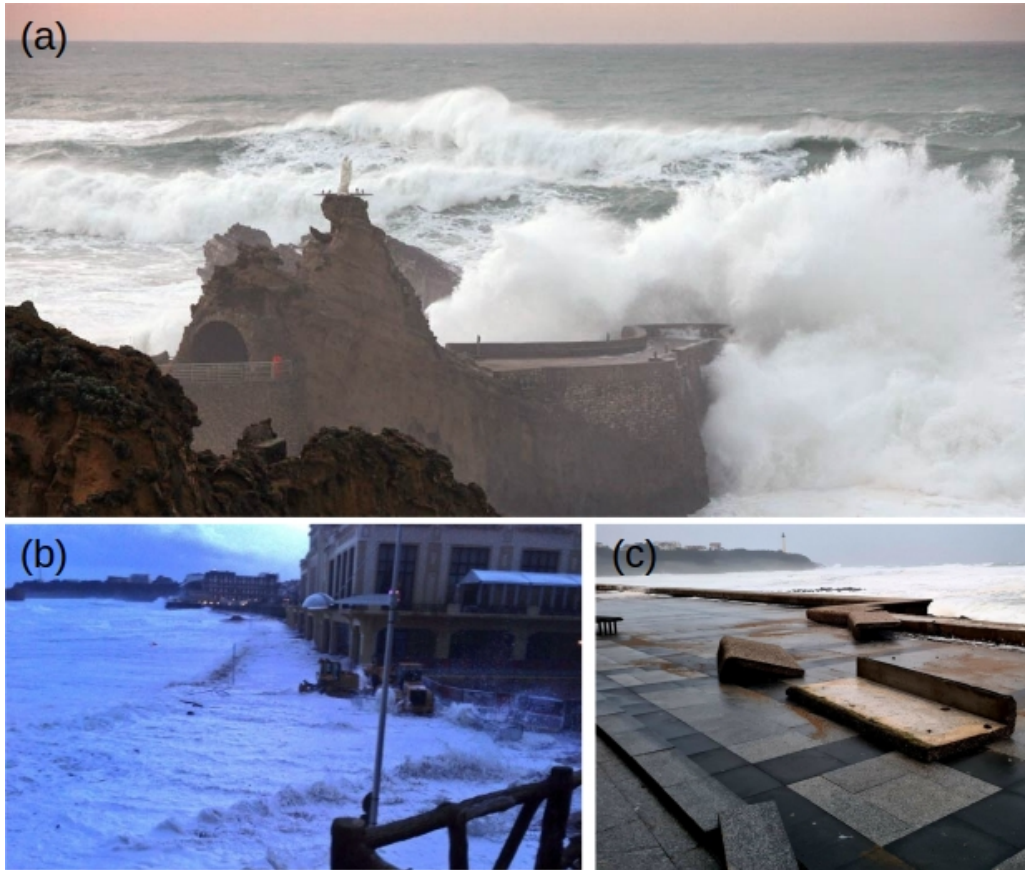
Figure 1.3: Storm impact along the Basque Coast. (a) Waves slamming the Rocher de la Vierge , © Isabelle Palé, (b) waves overtopping the seawall at the Grande Plage of Biarritz during the Hercules storm in 2014 © De Maria, (c) damaged sea wall at Anglet after the Justine storm of 2021 © Kty64.
