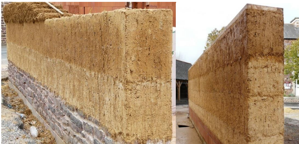
Figure 1-5 Cob wall construction [102]
