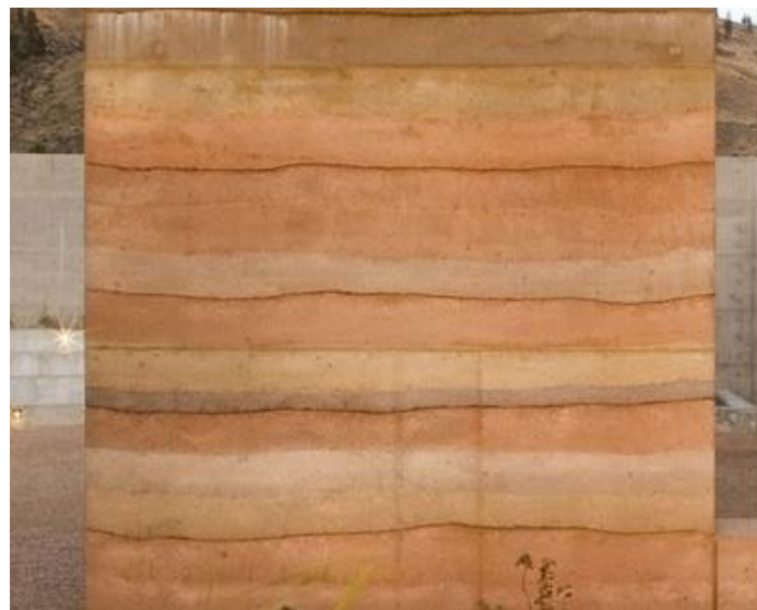
Figure 1-7 Rammed-earth construction [107]
