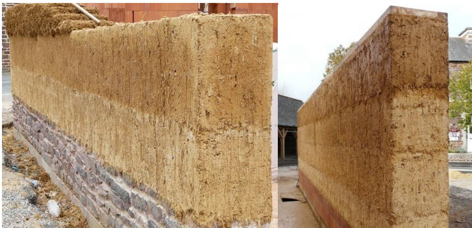
Figure 1-5 Cob wall construction [102]
