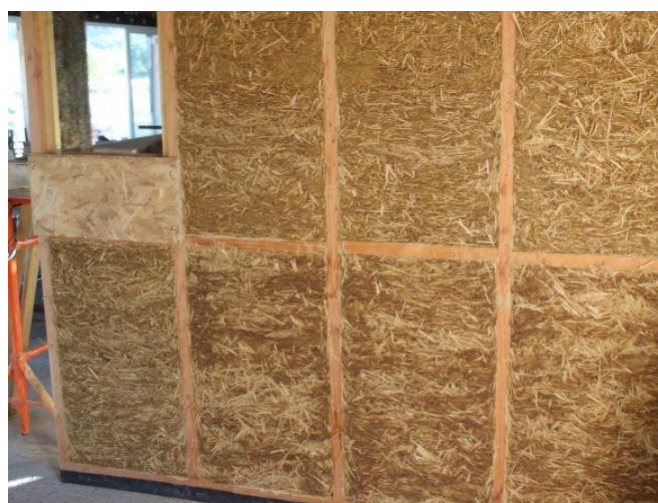
Figure 1-10 Lightened earth wall [110]
