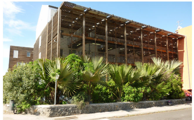
Fig. 1. Overview of the North facade of the case study: green patio with large solar protections.
