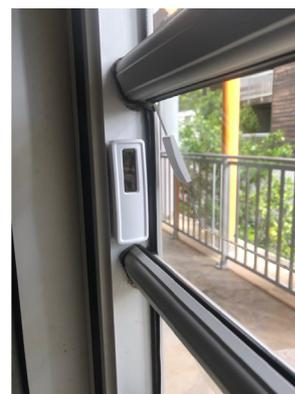
Fig. 3. Opened window (called louvers) with magnetic contact.
