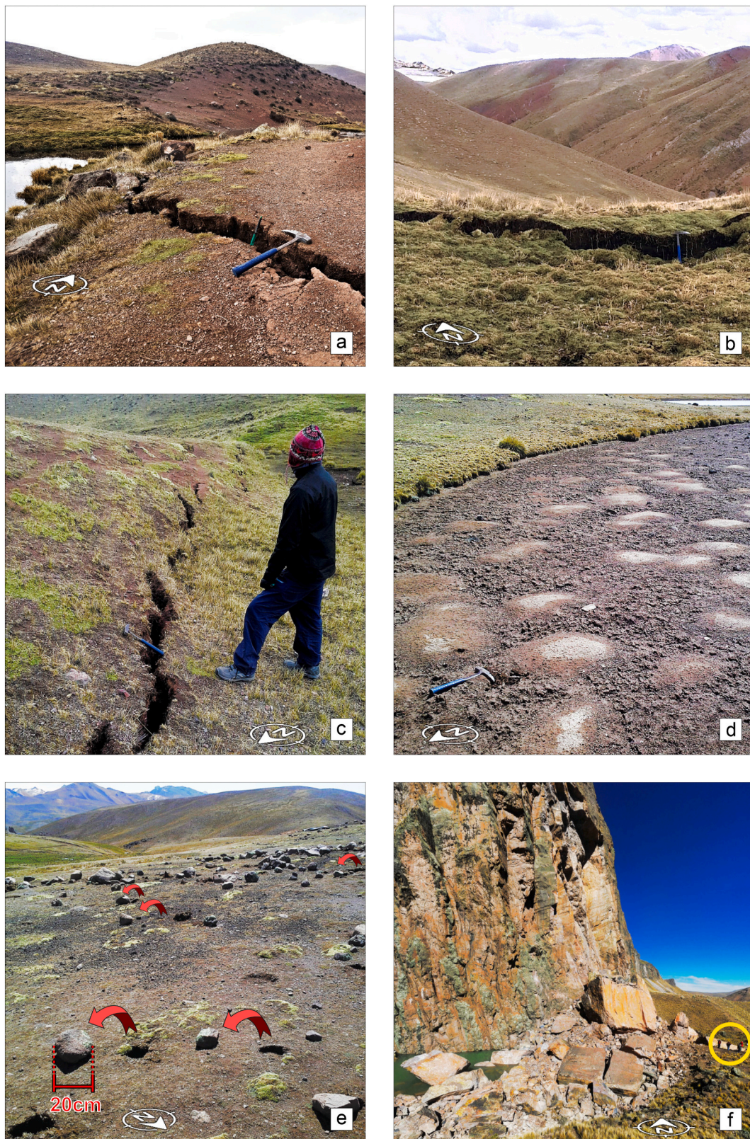
Fig. 4. Field photographs of coseismic surface ruptures and associated shaking effects. a) ~10 cm surface rupture, located in Lurini segment. b) ~27 cm surface rupture, located in Lurini segment. c) ~20 cm crack opening, located in Lurini segment. d) Sand boils west of the lake in Parina segment. e) Jumping stones, which are co-located with the sand boils, in Parina segment. f) Rockfall, which dammed the Jatun Ayllu River, some 12 km north of the epicenter. Note that near to surface rupture there is no more rock fall, probably due to the limited relief. See the yellow circle for the scale. (For interpretation of the references to color in this figure legend, the reader is referred to the Web version of this article.)
