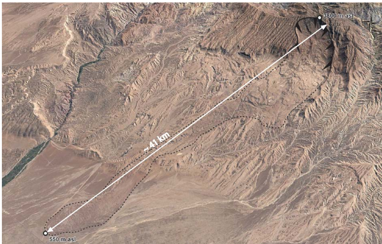
Figure 18. Caquilluco landslide (Rock avalanche). It has a drop between the headscarp and the foot of the landslide of ~3250 m and a strike length of ~41 km. Note that the landslide mass is preserved.
