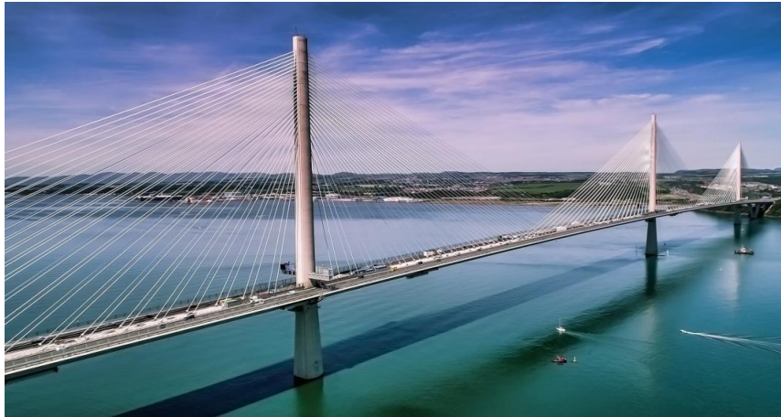
Figure 2.4: Photograph of the Queensferry Crossing a road bridge, in Scotland. With a length of 2.7 km, it incorporates about 37 km of pearlitic cabling, and it is the longest three-tower, cable stayed bridge in the world.
